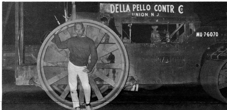
Kesky Sposs takes a whirl at street construction.
